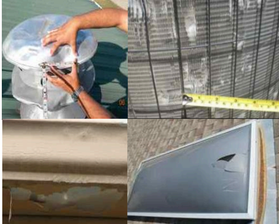
Figure 2. Examples of hail damage to non-structural components
