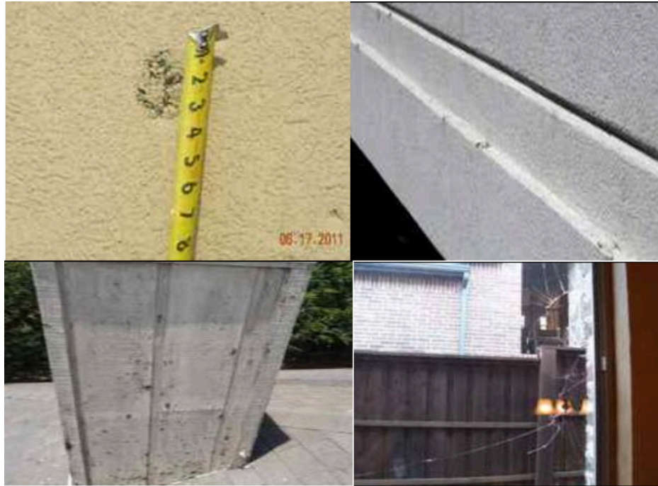
Figure 3. Examples of hail damage to wall siding and windows
