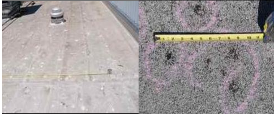
Figure 5. Examples of hail damage to roof covering
