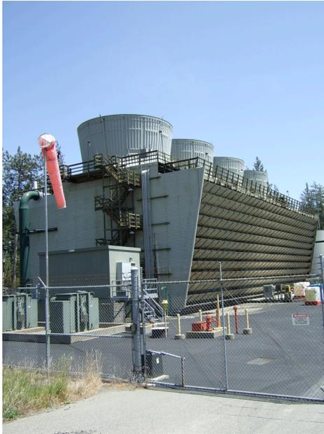
**Figure 147. West Ford Flat power plant geothermal cooling tower**
