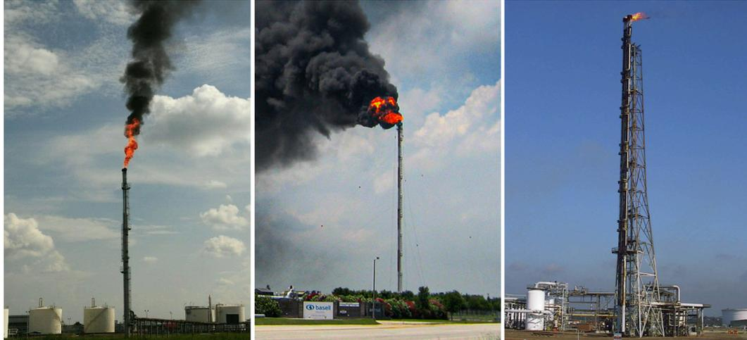
**Figure 149. Examples of flare tower types: freestanding (left), guyed flare (middle), and derrick-supported (right)**
