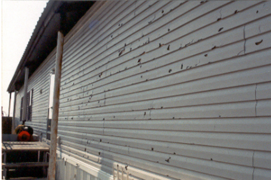
Figure 86. Hail damage to vinyl siding
