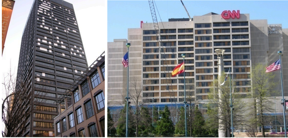
Figure 74. Tornado damage to much of the glass in commercial buildings in Atlanta, Georgia, on March 14, 2008 Source: Verisk
