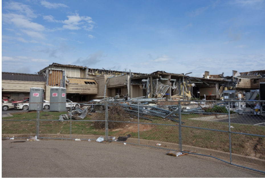
Figure 76. Tornado damage to a medical center in Moore, Oklahoma, on May 20, 2013 Source: Verisk
