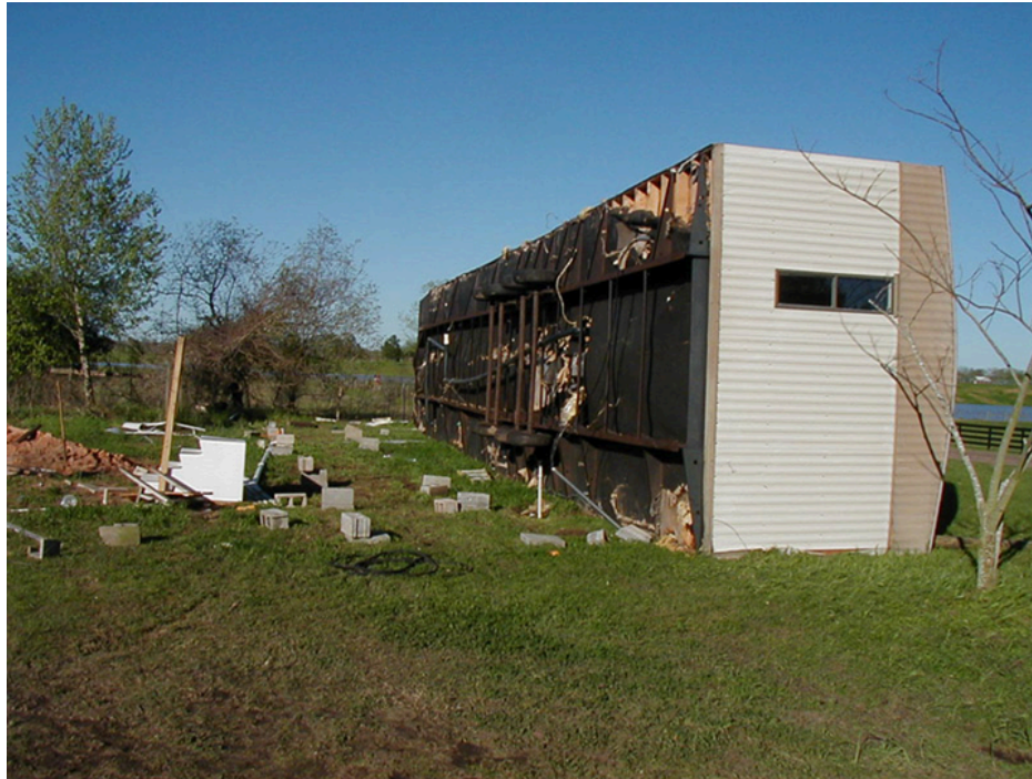
Figure 73. Significant straight-line wind damage to a manufactured home
