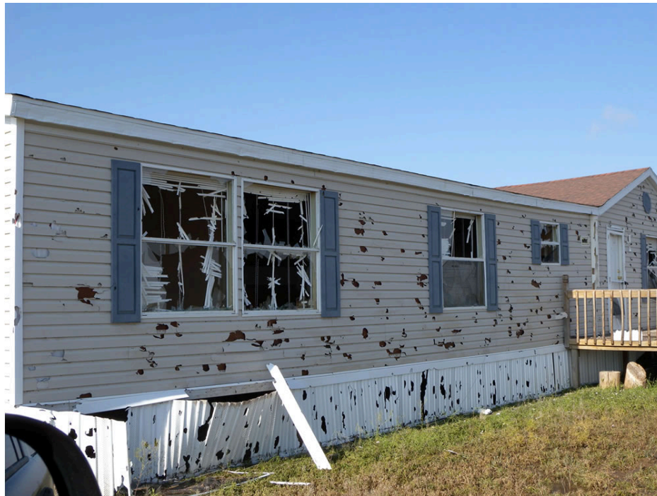
Figure 70. Significant hail damage to a manufactured home in Lubbock County, Texas Source: NOAA's National Weather Service
