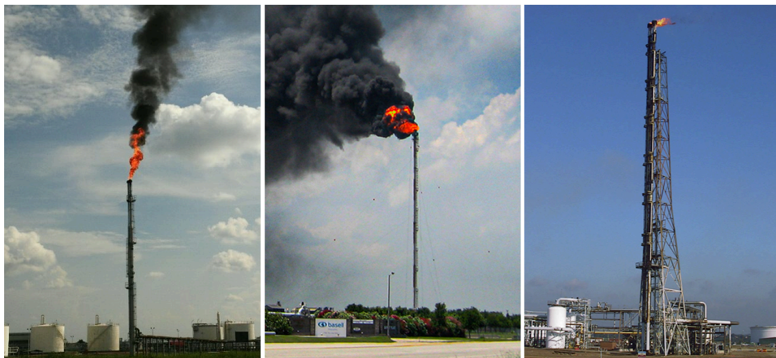
Figure 125. Examples of flare tower types: freestanding (left), guyed flare (middle), and derrick-supported (right)
