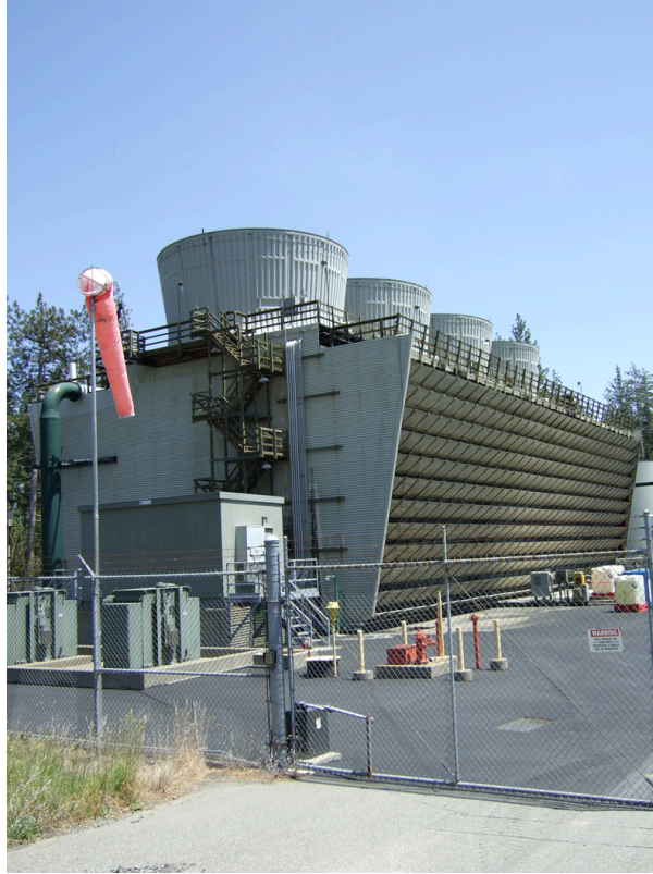
Figure 123. West Ford Flat power plant geothermal cooling tower
