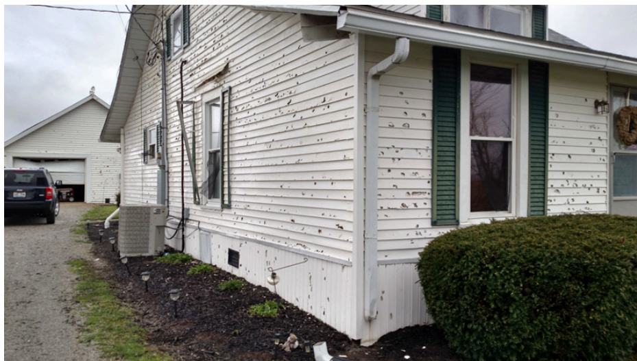
Figure 69. Significant hail damage to a single-family home
